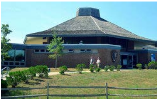
Salt Pond Visitor Center at Cape Cod National Seashore.
